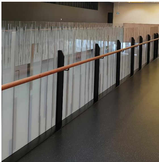
Figure 6.10: Sample of suitable balustrade
